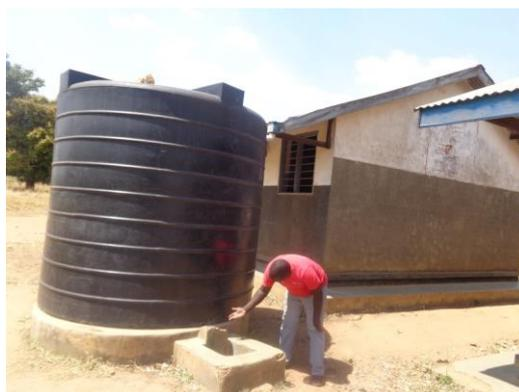
**Photograph 1. RWHT with missing tap and gutters**
