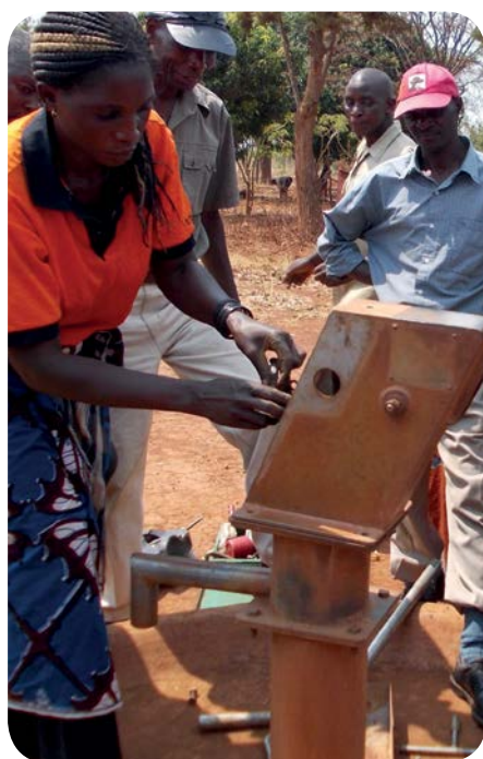
Pump mechanic in action, Zambia
