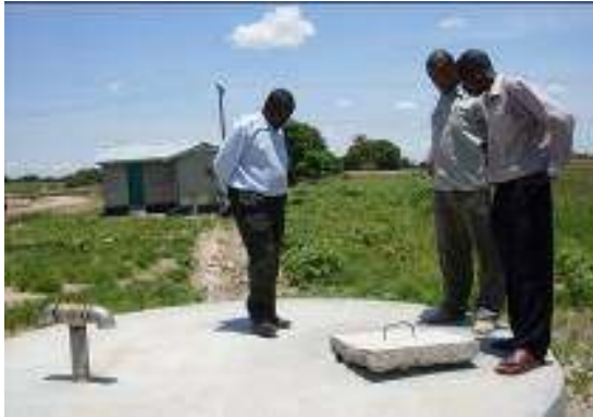
1. The Water Tank is Full
